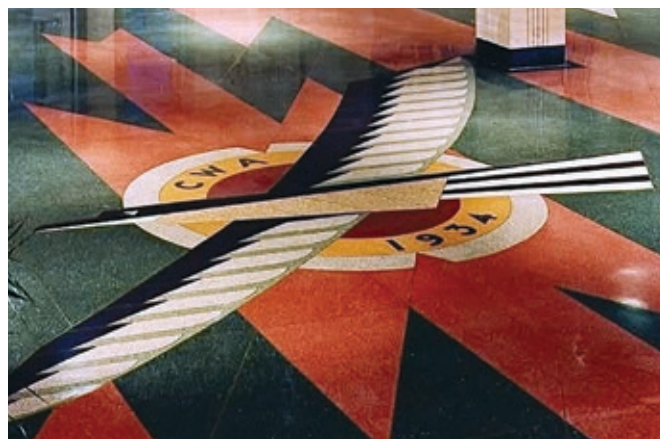
The terrazzo floor of the Building 1 lobby at EWR.
