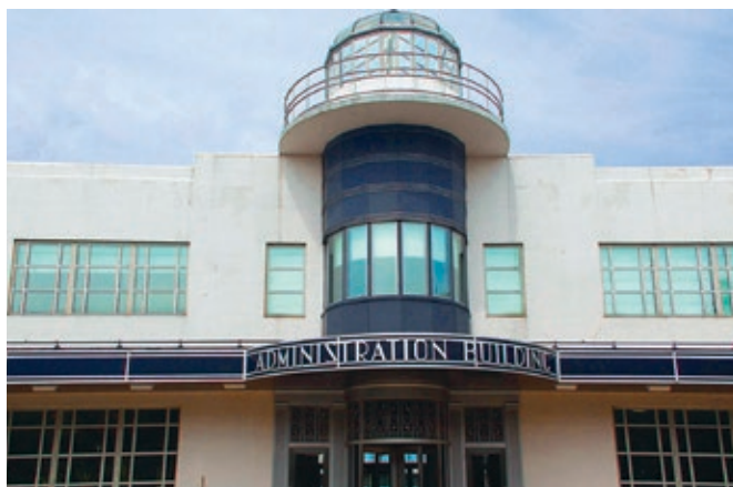
Building 1 at Newark Liberty International Airport.
