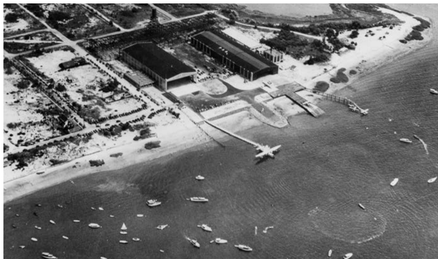
Aerial view of Pan American Airways hangars & launching docks, Port Washington Manhasset Bay 1938.
