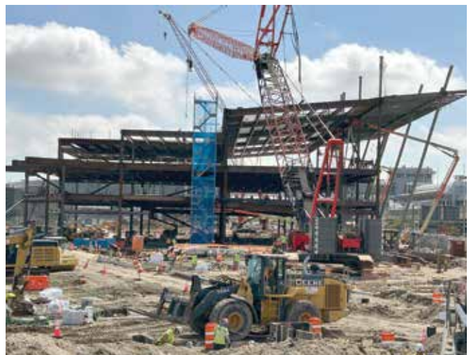
The structure of the new Terminal 6 becomes clearer each day.
