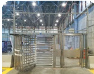
Access Control Systems JFK Airport
