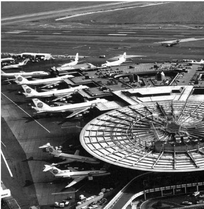
Pan Am's original terminal opened in 1960 and was extended the following decade.
